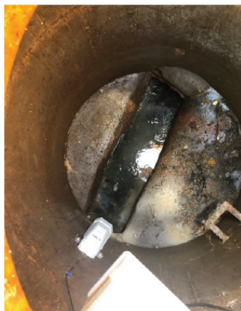
LIDoTT® Installed in a sealed sewer, with compression surcharge plate.
