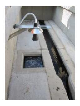
Level ONLY Flume (level sensor only controlling flow, lesser cost generally)
